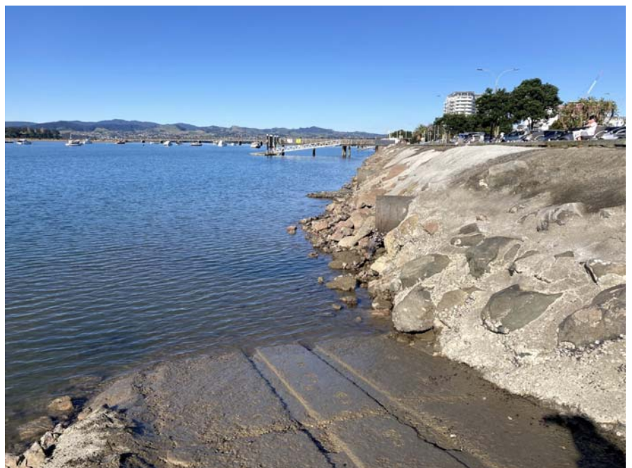
Figure 1: Existing seawall structure, June 2023 (Photo: WSP).
